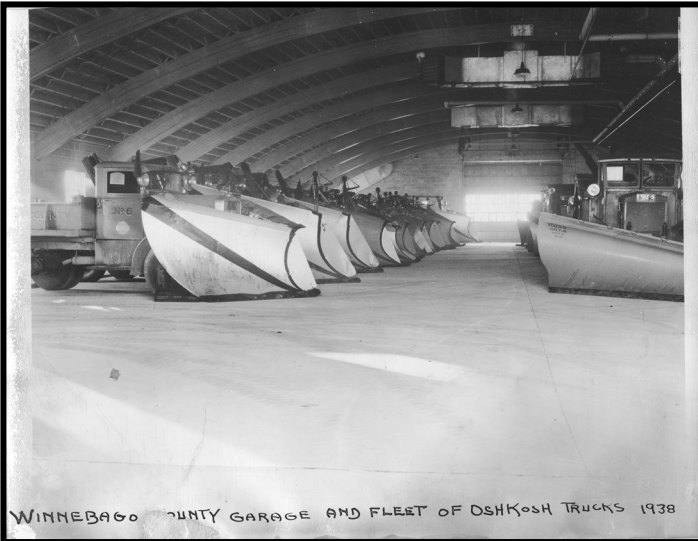
Highway garage interior - 1938 ( Courtesy of Winnebago County Highway Department )
