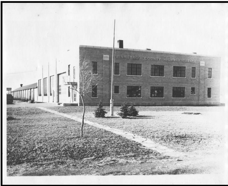
Winnebago County Highway Department repair shop addition - 1940 ( Courtesy of Winnebago County Highway Department )
